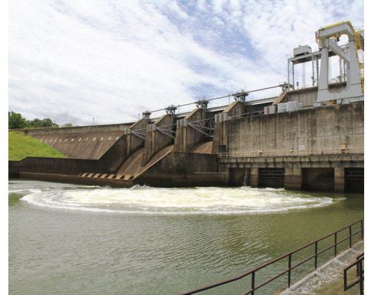
The Leesville, Va. dam supplies renewable power to Appalachian Power customers.
